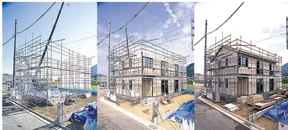
1) Construction of ground floor pillars and external walls.
