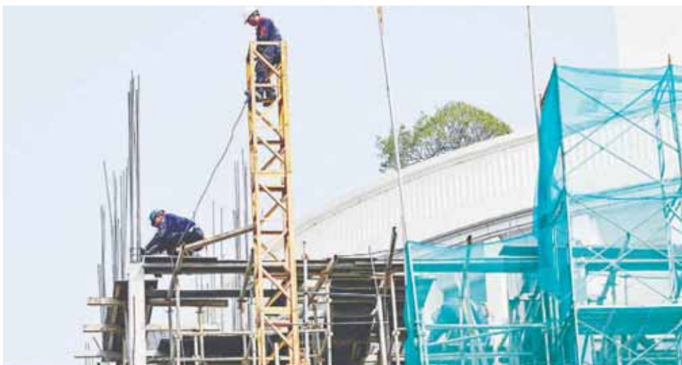
Workers standing on scaffolding at a construction site in Hanoi. – AFP/IC
