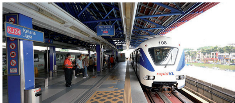
Kelana Jaya LRT station.
