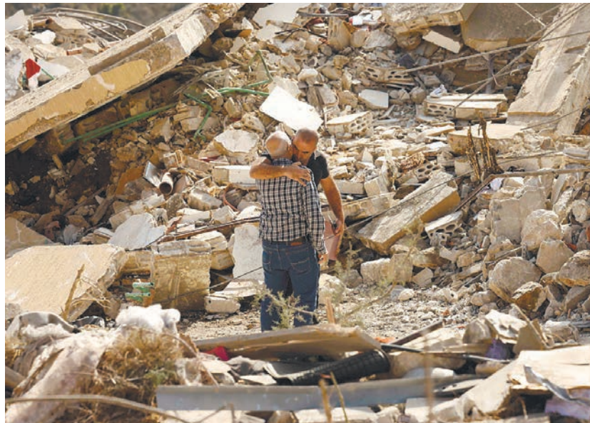
Affected residents console each other as they stand on the rubble of damaged buildings in the aftermath of Israeli strikes in Joun village in the Chouf district, Lebanon. - REUTERS/PIC
